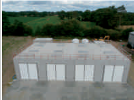
METHAJADE (France) 1 installation (55 kW)
